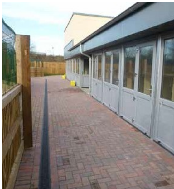
Safe area outside kennels and hard surfacing
